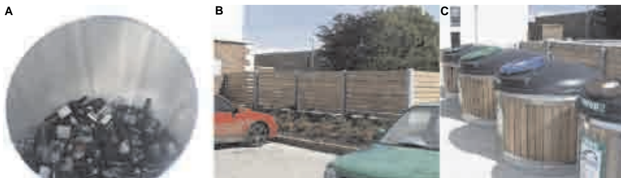
Figure 7.3. (A) Deep storage bottle bin. (B) Fenced-off waste storage area. (C) The four inlet bins.
