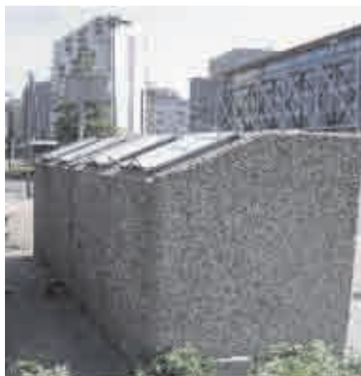
Figure 7.14. 240-l wheellie bins for organics and residual waste stored in concrete containers.
