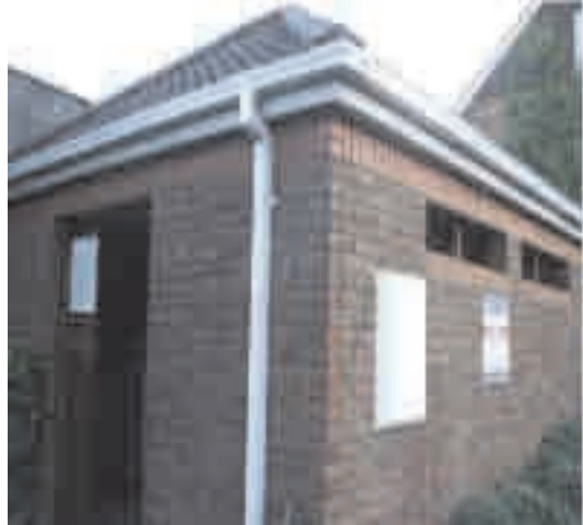
Figure 5.5. Designated bin storage shed.
