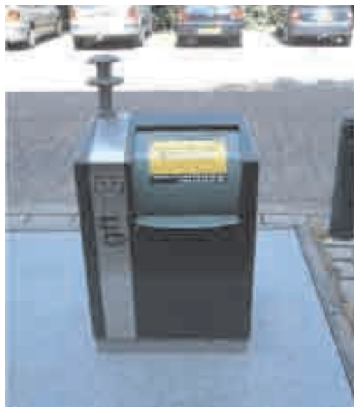
Figure 7.13. Bammens underground organic waste bins, 3,000 l.
