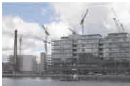
Figure 5.2. Apartment block construction.
